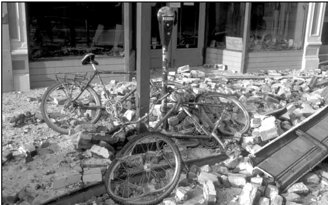
1989 Loma Prieta earthquake: Bicycles are crushed by falling unreinforced brick facade, Santa Cruz, Calif. PHOTO: U.S. Geological Survey
